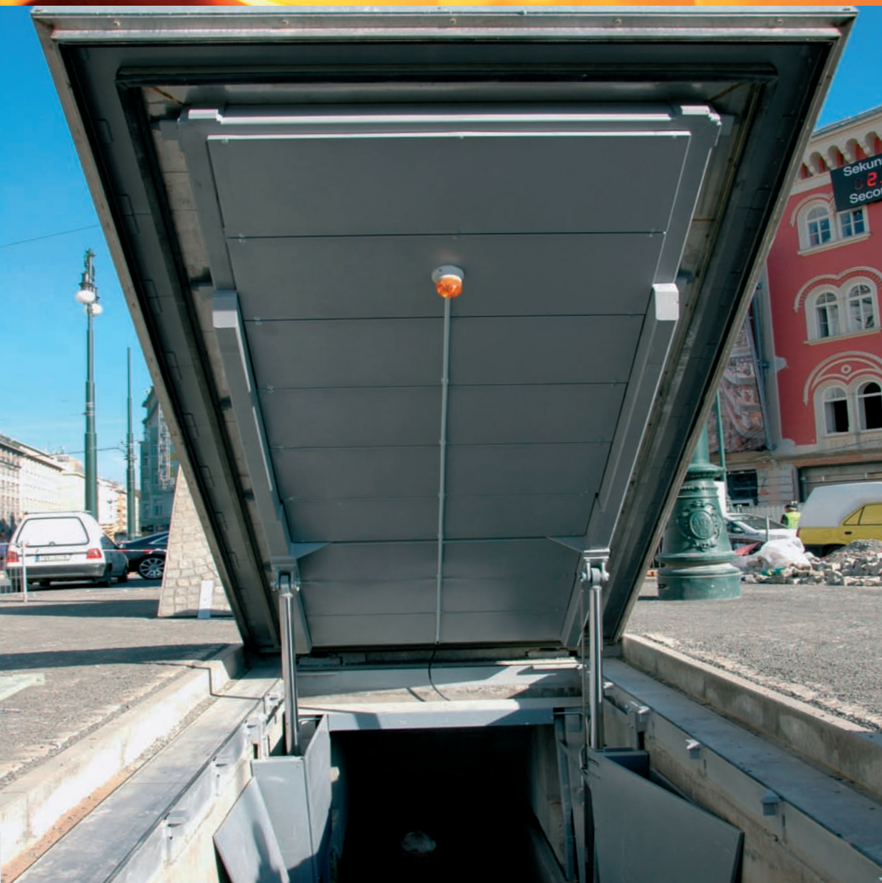
Escape cover 2500 x 5000 mm for an emergency escape of people in the case of fire; it is movable and fitted into the road of Náměstí Republiky Square in Prague as an exit of an escape underground corridor from three-floor underground garages. It opens automatically.
